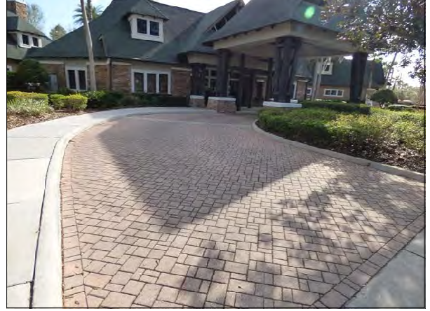
Amenity Center Parking Lot Pavers
