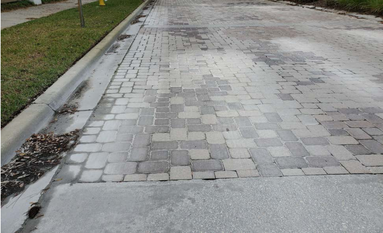
Brick Paver Repair #1 Photo
